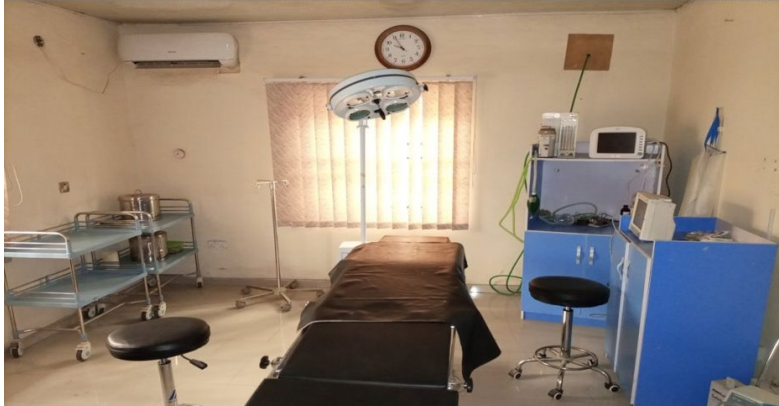
The above picture shows the operating room in the hospital. The operating theatre is one of the high priority departments at the facility to receive donations.
